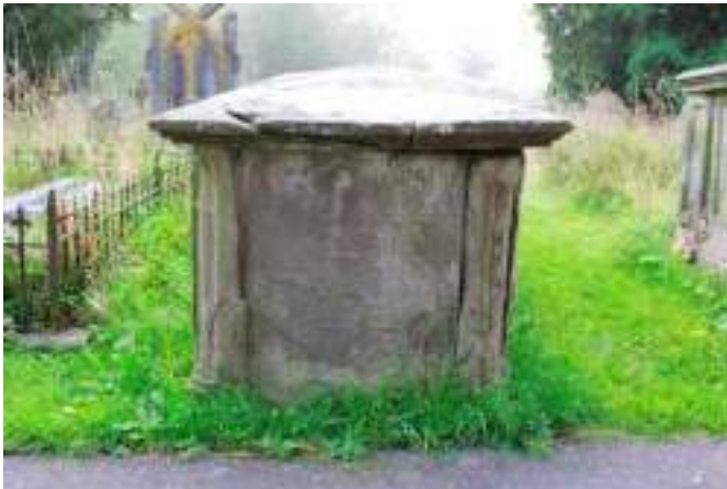
The west elevation of the memorial, highlighting subsidence in two planes east – west and north – south. The laminations in the lid can be seen more clearly in this image, largely attributable to the level of deformation witnessed in the underlying tomb chest.
