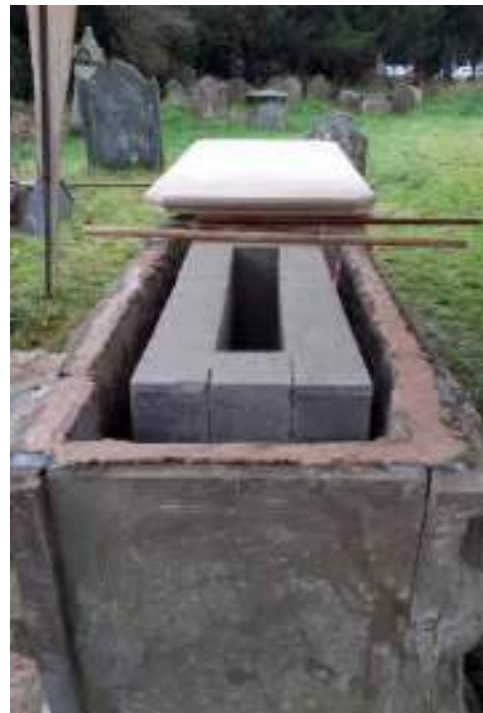
Fixing of the new Woodkirk - Sandstone (Building Quality as opposed to Monumental Quality) being slid into position. The small amount of bedding mortar on the top-bed of the plinth is to give something solid against which the gunnable pointing mortar can be forced against, thus ensuring a solid joint from back to front, which is not achievable when just pointing from the front face using a traditional, coarse mortar. There was no need to secure the tomb chest panels back to the core as the fixings between themselves were so solid. The original lid appeared to have been completely flat, shallow angled 'weatherings' were incorporated into the new slab to shed rainwater more effectively and prevent water pooling on the surface.
