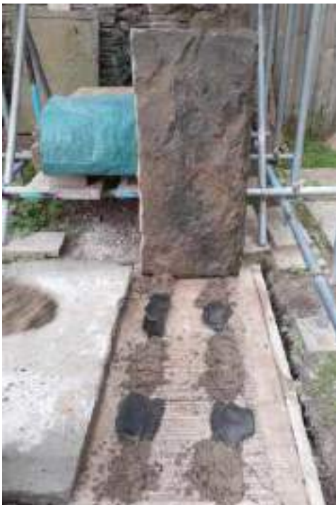
The newly joined section before bedding on mortar and slate packers. The whole perimeter was deep-tamped with mortar. Once this had hardened sufficiently liquid grout (based on NHL3.5) was introduced into the joint from front to back, to provide additional support once hardened.
