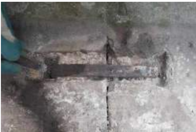
The turn-downs were filled with lime mortar, which is a soft material anyway but didn't stand a chance once excess water had got in and was allowed to sit there, due to defective pointing. The fixings were simply lifted out with a chisel. The central joint was stoned to stone and it shouldn't be. We used new stainless-steel cramps secured with epoxy-resin and lead shims in the central joint, so the blocks can't move again.
