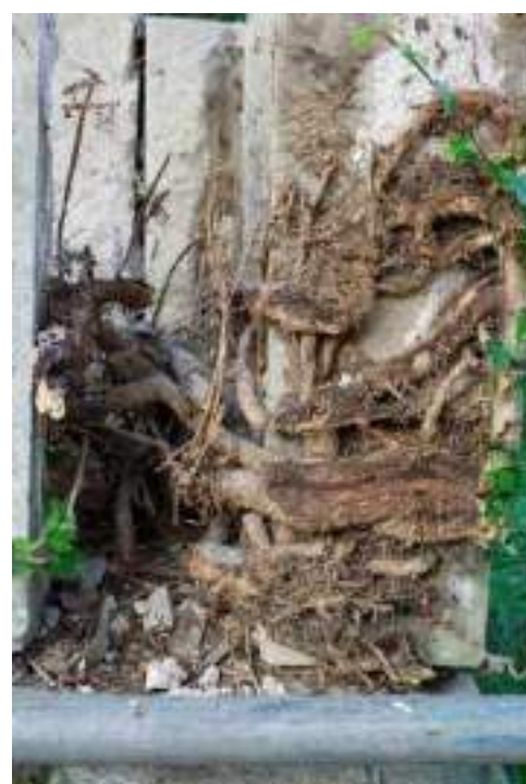
Detail of disruption over two courses, forcing significantly heavy blocks apart and breaking fixings (albeit corroded) apart. On the right, after removal of one of the corner blocks showing how the stems are compressed in the joint but still able to exert enormous, damaging forces over time.
