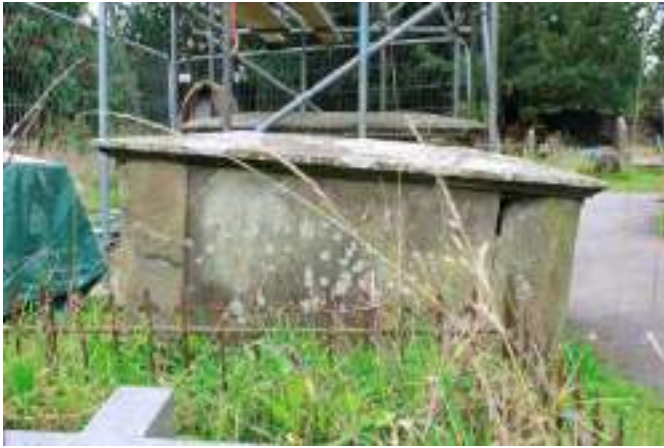
The extent of subsidence prior to dismantling. Note again the proximity of the nearby path and adjacent railings.
