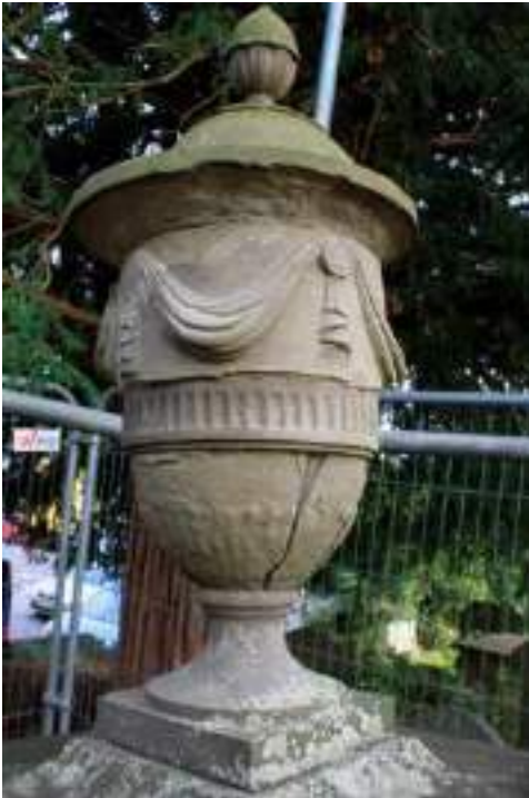
On the left, the urn prior to dismantling, note the lid above the swag or draped layer is loose and could have been dislodged in high winds, causing damage to these carved elements. On the right, the top-bed of the diminishing lower-urn during removal of the expanded iron-dowel. The existing fracture, both sides were full of organic debris and insects.
