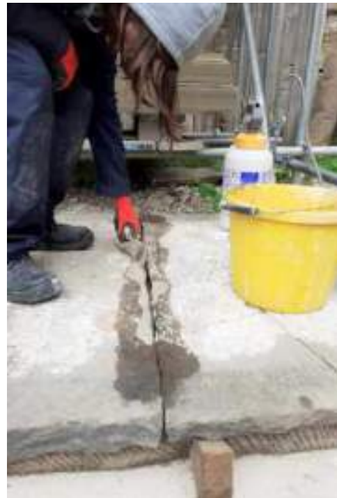
The newly joined section before bedding on mortar and slate packers. The whole perimeter was deep-tamped with mortar. Once this had hardened sufficiently liquid grout (based on NHL3.5) was introduced into the joint from front to back, to provide additional support once hardened.
