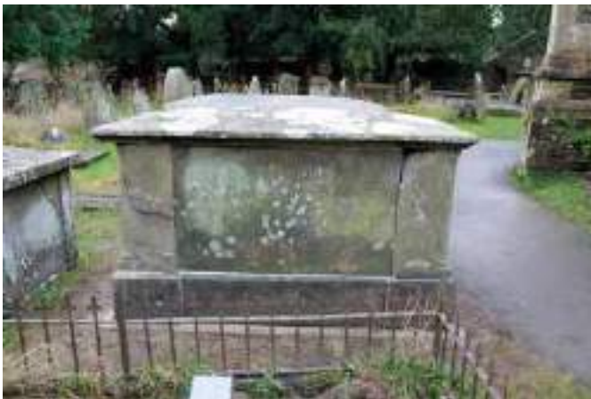
The memorial after nearly all treatments. Note the concrete sub-base is just below ground level and the path but the void between both is filled with free-draining aggregate, which will prevent water pooling in this location. The plinth will dry slowly in time, having been below ground-level for so long.
