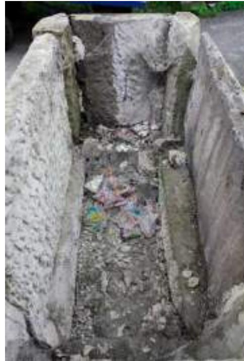
The tomb chest once the lid was removed. On the left, note the thin nature of the bedding surface (indicated) the rear of which slopes away, leaving only 10-15mm of bearing. On the right, detritus on the inside of the chest. The west elevation, 'short' side shows where (white) liquid plaster has been poured in historically, in a vain attempt at consolidation.
