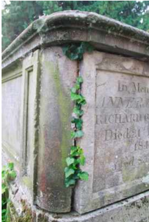
On the left, the north-west corner block being forced out, despite point-loading along the north elevation. On the right, the south-east corner block with its now very dove-tailed joint caused by ivy growth. The joint should be as it is at the top, instead of widening significantly towards the bottom-bed.
