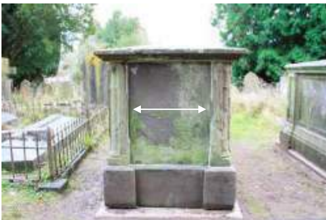
The west elevation of the memorial showing the relation between the neighbouring kerb set/railings and Griffiths memorial to the right. The gap between the two memorials is a mown path and we didn't want to create a trip-hazard on the corners of either sub-base. Note the inner mouldings or rebates on the two, rounded corner-blocks (indicated) is largely missing and why the joints look so wide.
