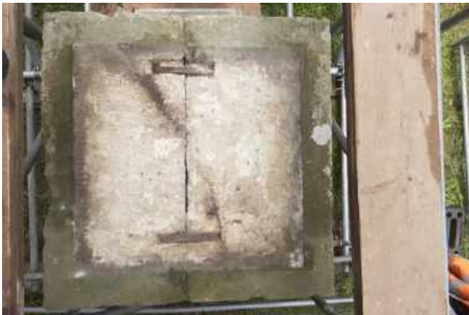
After brushing to removed defective bedding mortar and debris. The two fixings have failed, allowing the joint to collapse in on itself. It would have been better to include slate in the joint so they couldn't rotate, causing the point-loading they did, in the 'short' box-panels.
