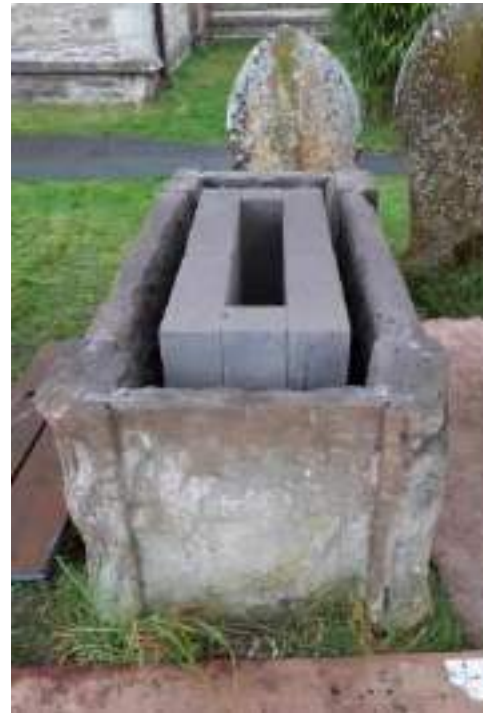
Building of the core in progress, using Celfix® mortar to create tight, uniform joints. The completed core in the right image. The top-bed of the core was built too high for the tomb chest elements (intentionally) and 'dragged' back to give the correct height and uniform joint between the tomb chest and new lid.
