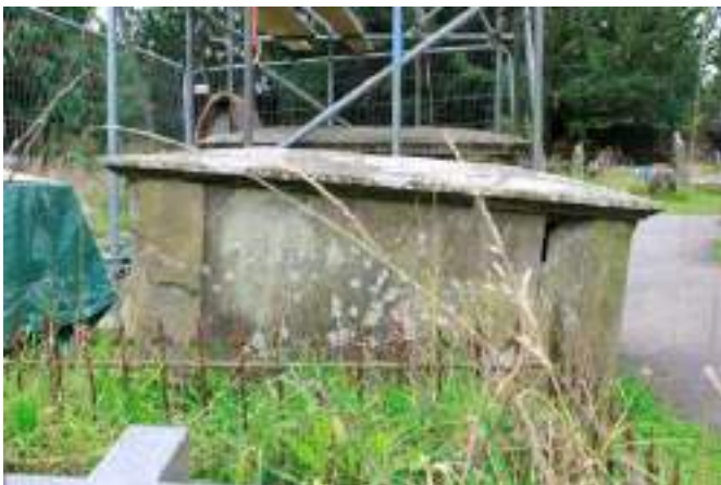
The north elevation of the memorial highlighting the extent of subsidence and the proximity of the path. The iron railings in the foreground are more or less level across their top.
