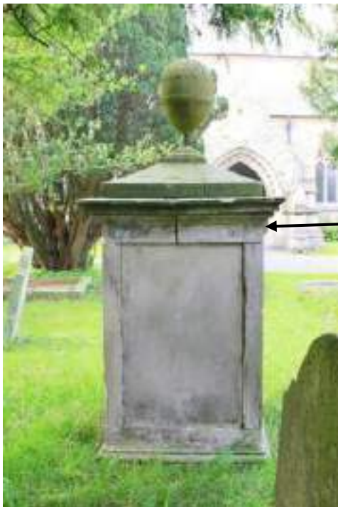
The rear, north elevation before (left) and after all treatments. Note how the moulded entablature (indicated) shows a dovetailed, vertical, central-joint, due to failed fixings - causing point-loading on the 'short' box panels beneath, at the front and back. That situation was significant on this elevation, contributing to the inside of the panel delaminating in half and being substantially weaker as a result. The resultant joints lines have all been pointed from back to front, with a fluid, gunnable mortar.
