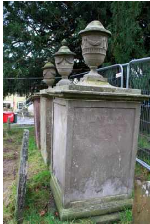
The south elevation of the memorial to William & Ann Hughes before and after all treatments. Note the parallel joint between the capstone and the box-panels, pointed on the right image. The shallow, moulded plinth and sub-base is just visible through the grass on this elevation.
