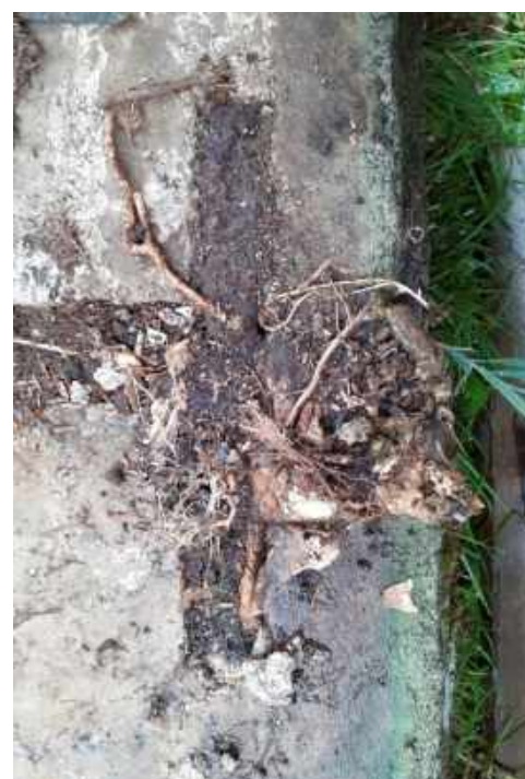
Corroded iron fixings which have delaminated to now flaky metal, serving no useful purpose. Luckily there was no iron-staining to speak of, despite there being easy access for excess moisture, with which to initiate the process. On the right, ivy stems grow easily beneath the fixing, ready to force this one apart.
