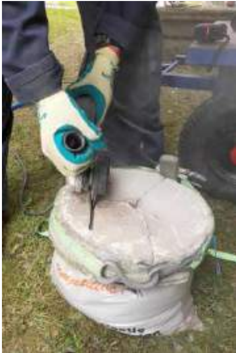
Slots being ground into the urn and afterwards with the flat-bar set-in with the now hard, external grade epoxy-resin.
