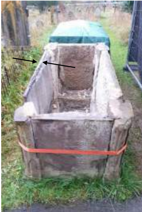
The tomb chest once the lid was removed. On the left, note the thin nature of the bedding surface (indicated) the rear of which slopes away, leaving only 10-15mm of bearing. On the right, detritus on the inside of the chest. The west elevation, 'short' side shows where (white) liquid plaster has been poured in historically, in a vain attempt at consolidation.
