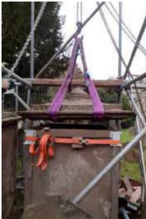
Once the urn was removed, which was also lifted using the block and tackle given its combined weight, the capstone and urn-base was raised slightly, moved horizontally on the girder-trolley before lowering onto the turn-table truck below and away from the area of work. Note the very uneven nature of the bottom-bed of the capstone, with the surface having a rough 'punched' finish from the workshop.
