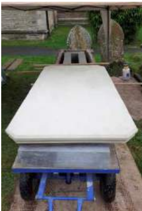
Fixing of the new Woodkirk - Sandstone (Building Quality as opposed to Monumental Quality) being slid into position. The small amount of bedding mortar on the top-bed of the plinth is to give something solid against which the gunnable pointing mortar can be forced against, thus ensuring a solid joint from back to front, which is not achievable when just pointing from the front face using a traditional, coarse mortar. There was no need to secure the tomb chest panels back to the core as the fixings between themselves were so solid. The original lid appeared to have been completely flat, shallow angled 'weatherings' were incorporated into the new slab to shed rainwater more effectively and prevent water pooling on the surface.
