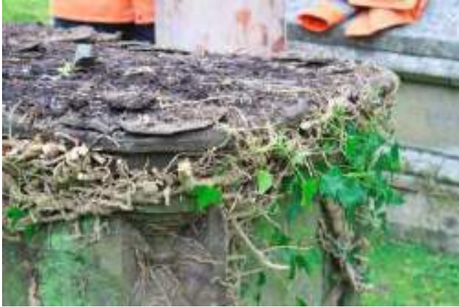
During removal of ivy growths, which couldn't be removed properly until the tomb chest was dismantled fully. Note the extent of soil debris on the top-bed of the slab from the breakdown of ivy-leaves over many years.
