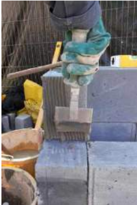
Building of the core in progress, using Celfix® mortar to create tight, uniform joints. The completed core in the right image. The top-bed of the core was built too high for the tomb chest elements (intentionally) and 'dragged' back to give the correct height and uniform joint between the tomb chest and new lid.
