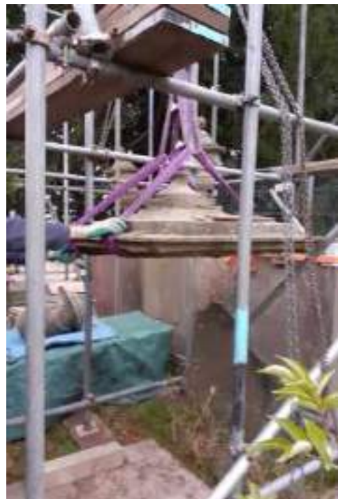
Once the urn was removed, which was also lifted using the block and tackle given its combined weight, the capstone and urn-base was raised slightly, moved horizontally on the girder-trolley before lowering onto the turn-table truck below and away from the area of work. Note the very uneven nature of the bottom-bed of the capstone, with the surface having a rough 'punched' finish from the workshop.
