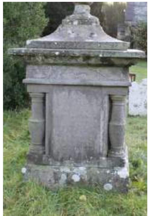
The west elevation of the Thomas memorial before and after all treatments. Delaminated stone along the bottom bed of this elevation was also rationalised back to sound substrate, with support fillings inserted along the length of the previously tacked edges. Carved detail to the frieze is a little easier to determine on this elevation.
