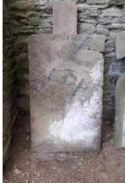
The front (viewer's left-hand side) and the rear (right-hand side) of the same panel showing the number of mechanical fixings to provide additional support in the side-to-side fractures. The slab was too thin to insert dowels in the centre, so 12 x 3mm stainless-steel flat-bar is inserted at right-angles across fractures, into cut channels and secured with epoxy-resin. The panel is upside down and stayed that way until re-building, so as not to stress the two horizontal joins unnecessarily, which could have failed given the overall weight/height of the slab.
