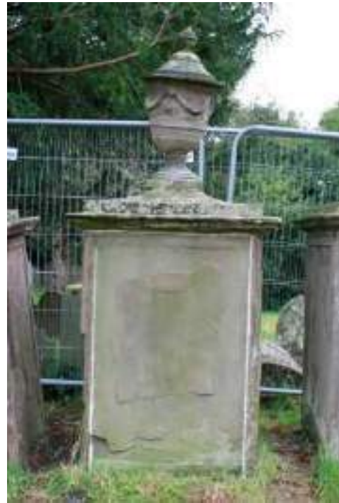
The memorial to Mary Hughes before and after all treatments. On the left, the Yew tree branches brushing the urn, prior to being pruned back. The box panel on this elevation was actively loose when the capstone and urn were lifted off. The new pointing mortar is the same colour as the original fat-lime mix.
