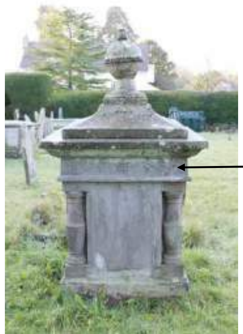
The north elevation of the Thomas memorial before and after all treatments. Delaminated stone along the bottom bed of the box-tomb was rationalised back to sound substrate, with support fillings inserted along the length of the previously tacked edges. Note the poor angle of the ball-finial. Low-relief, foliate-decoration to the frieze (indicated) beneath the capstone is all but lost visually.
