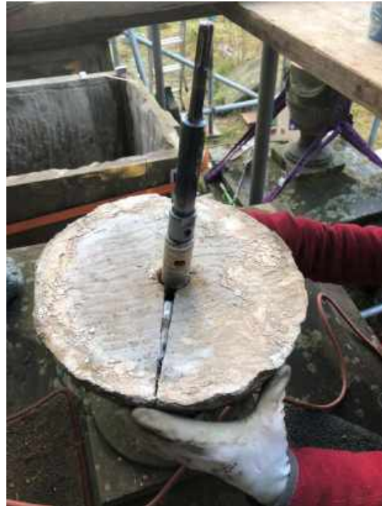
On the left, the urn prior to dismantling, note the lid above the swag or draped layer is loose and could have been dislodged in high winds, causing damage to these carved elements. On the right, the top-bed of the diminishing lower-urn during removal of the expanded iron-dowel. The existing fracture, both sides were full of organic debris and insects.
