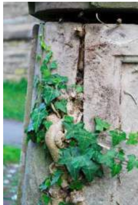
On the left, the north-west corner block being forced out, despite point-loading along the north elevation. On the right, the south-east corner block with its now very dove-tailed joint caused by ivy growth. The joint should be as it is at the top, instead of widening significantly towards the bottom-bed.
