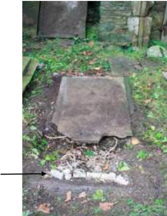
The bottom side panel with fractured elements safely removed. Note the remains of very thick white mortar (indicated) which formed a joint between the bottom bed of the inscription panel and top bed of the plinth which you can just see beneath ground level. This indicates an overly wide joint, due to structural instability. The right-hand image shows some of the elements leaning against a nearby wall, to be rain-washed over the winter and the capstone and urn moved away to one side, to enable erection of a lifting scaffold.
