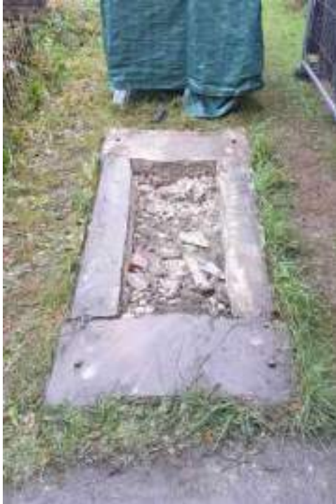
On the left the plinth showing how much subsidence has taken place and how much the churchyard has risen over the 186 years since it was likely built. On the right, the plinth blocks have been moved. There were only two re-cycled tomb chest slabs at the far, east end, providing any sort of sub-base. Note the proximity of the railings and underlying kerb-set to the north.
