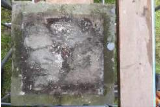
The top-bed of the entablature after removal of the capstone. Note the amount of debris in there, which is introduced by water, from defective/empty joints due to lack of maintenance.
