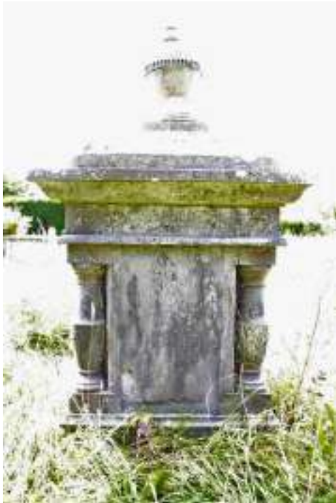
The north elevation of the Thomas memorial before and after all treatments. Delaminated stone along the bottom bed of the box-tomb was rationalised back to sound substrate, with support fillings inserted along the length of the previously tacked edges. Note the poor angle of the ball-finial. Low-relief, foliate-decoration to the frieze (indicated) beneath the capstone is all but lost visually.
