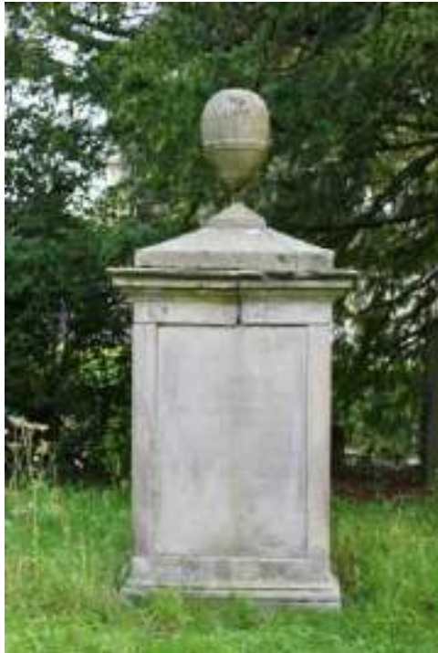
The memorial to William Thomas before (left) and after treatments. Outwardly there appears to be very little difference, however before treatment the memorial could have been pushed-over with a concerted effort, given its top-heavy design and failure of corroded iron-fixings. Note the greater level of colonisation with black biological growths to the ovoid ball-finial between July and December. No cleaning took place on this object.
