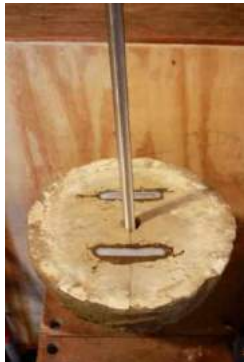
On the left, after removal of the fractured lower section, see how the delaminating iron-dowel had expanded into the available space before forcing the stone apart, exerting huge pressure to split the block. On the right, the repaired lower urn section with new, threaded stainless-steel dowel issuing from the top. The drill-hole between the steel (which cannot corrode) was filled with a pourable anchor grout used in civil engineering.
