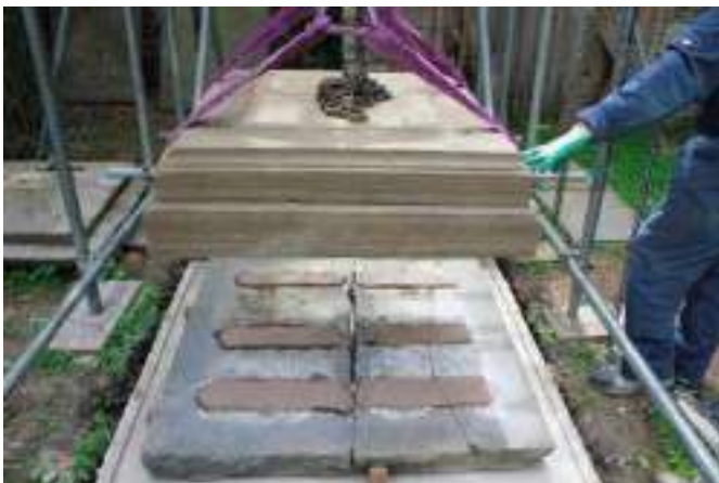
The moulded plinth being lowered into position. The girder-trolley above, allowed exact placement of this heavy section, without need for adjustments when grounded and disrupting the mortar bed.
