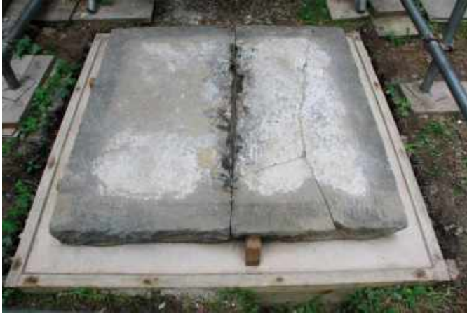
The repaired sub-base with preliminary pointing and grouting completed.
