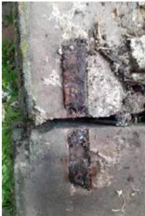
Corroded iron fixings which have delaminated to now flaky metal, serving no useful purpose. Luckily there was no iron-staining to speak of, despite there being easy access for excess moisture, with which to initiate the process. On the right, ivy stems grow easily beneath the fixing, ready to force this one apart.
