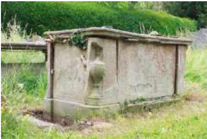
After removal of the surface growths, with stems still growing through the joints. Note the upward plane of the tomb chest lid in the foreground and the horizontal fracture through the slab as a result.
