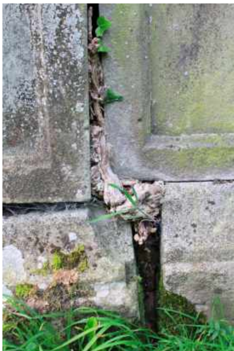
Detail of disruption over two courses, forcing significantly heavy blocks apart and breaking fixings (albeit corroded) apart. On the right, after removal of one of the corner blocks showing how the stems are compressed in the joint but still able to exert enormous, damaging forces over time.
