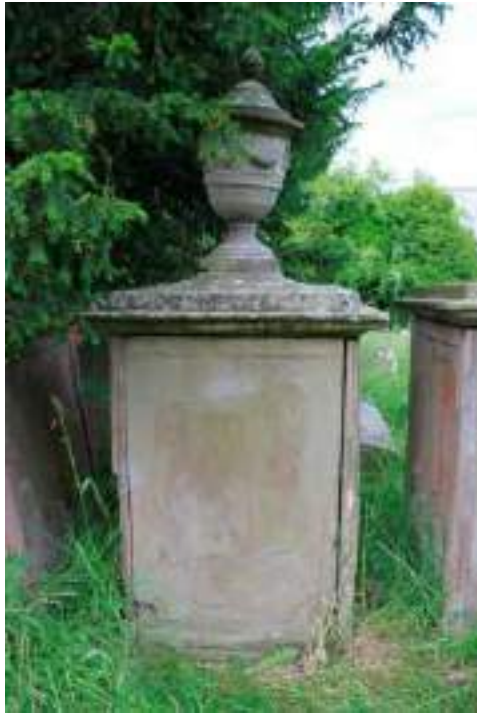
The memorial to Mary Hughes before and after all treatments. On the left, the Yew tree branches brushing the urn, prior to being pruned back. The box panel on this elevation was actively loose when the capstone and urn were lifted off. The new pointing mortar is the same colour as the original fat-lime mix.
