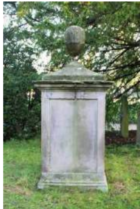
The memorial to William Thomas before (left) and after treatments. Outwardly there appears to be very little difference, however before treatment the memorial could have been pushed-over with a concerted effort, given its top-heavy design and failure of corroded iron-fixings. Note the greater level of colonisation with black biological growths to the ovoid ball-finial between July and December. No cleaning took place on this object.
