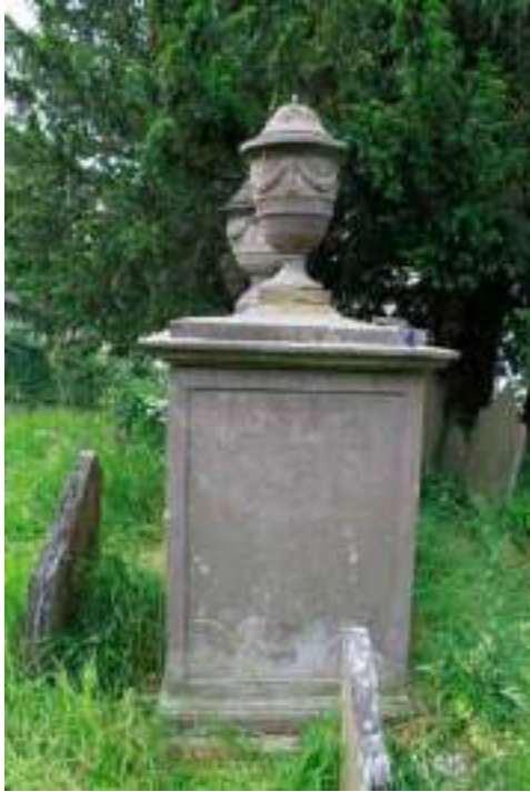
The south elevation of the memorial to William & Ann Hughes before and after all treatments. Note the parallel joint between the capstone and the box-panels, pointed on the right image. The shallow, moulded plinth and sub-base is just visible through the grass on this elevation.
