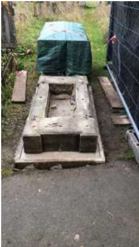
On the left the new re-enforced sub-base in position with the plinth blocks having been bedded into position. On the right, the void within the plinth has been filled with Limecrete, on top of a Visqueen DPM/separation layer. Celcon blocks being laid to create a supporting internal core.
