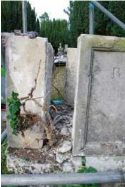
On the left, the south-west corner block having been removed, showing the stems continuing down into the next course. Note how there is no bedding in the bottom-bed of the tomb chest panels. On the right, the south-east corner showing the substantial fixing has been pulled apart with the corroded turn-down, left in the left-hand socket. The joint should be 5mm wide not 30mm
